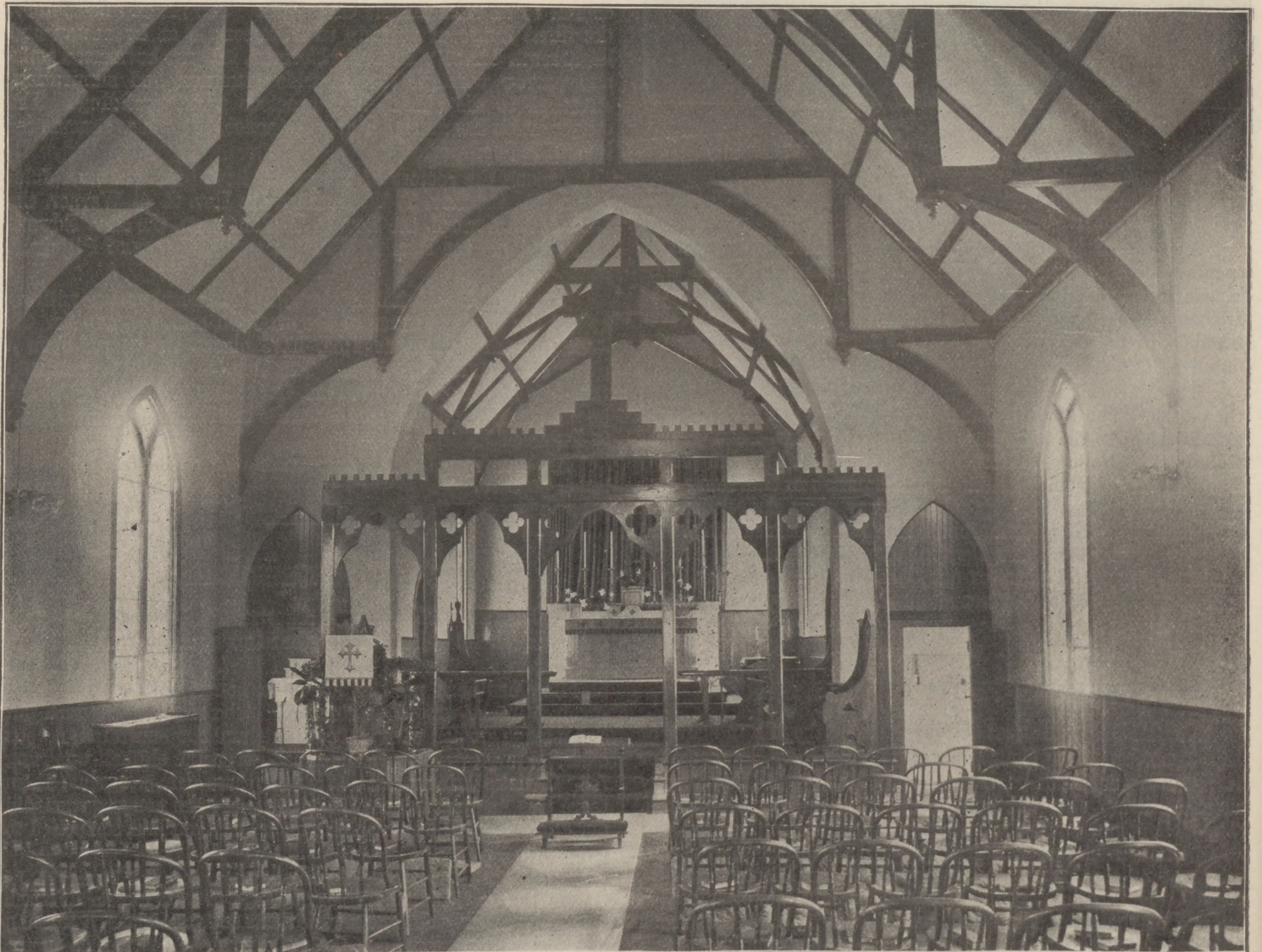
ST. JAMES' CHURCH (AS RESTORED), HACKETTSTOWN, N. J.
