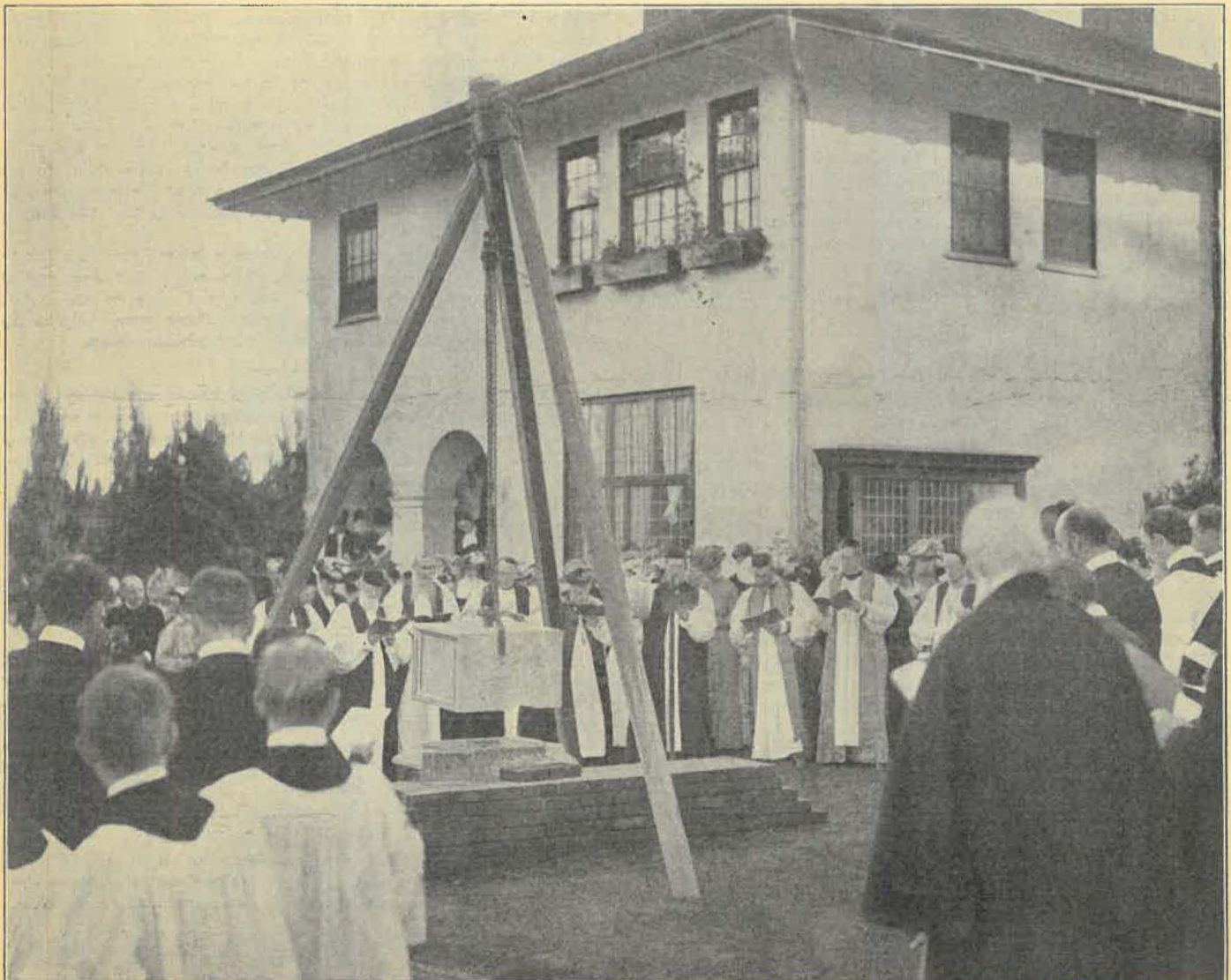
LAYING OF THE CORNER-STONE—CHAPEL OF THE CHURCH DIVINITY SCHOOL, SAN MATEO, CAL.
