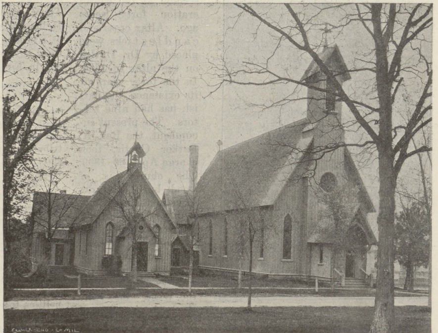
ST. PETER'S CHURCH, RIPON, WIS.
