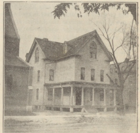
ARMITAGE HOUSE. PRESBYTERY OF ALL SAINTS' CATHEDRAL, MILWAUKEE.
