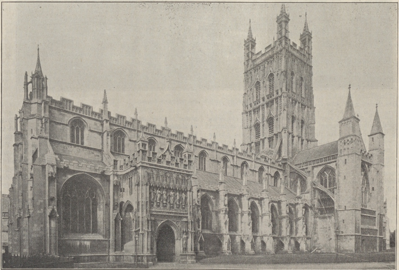
GLOUCESTER CATHEDRAL—VIEW FROM THE SOUTHWEST.
