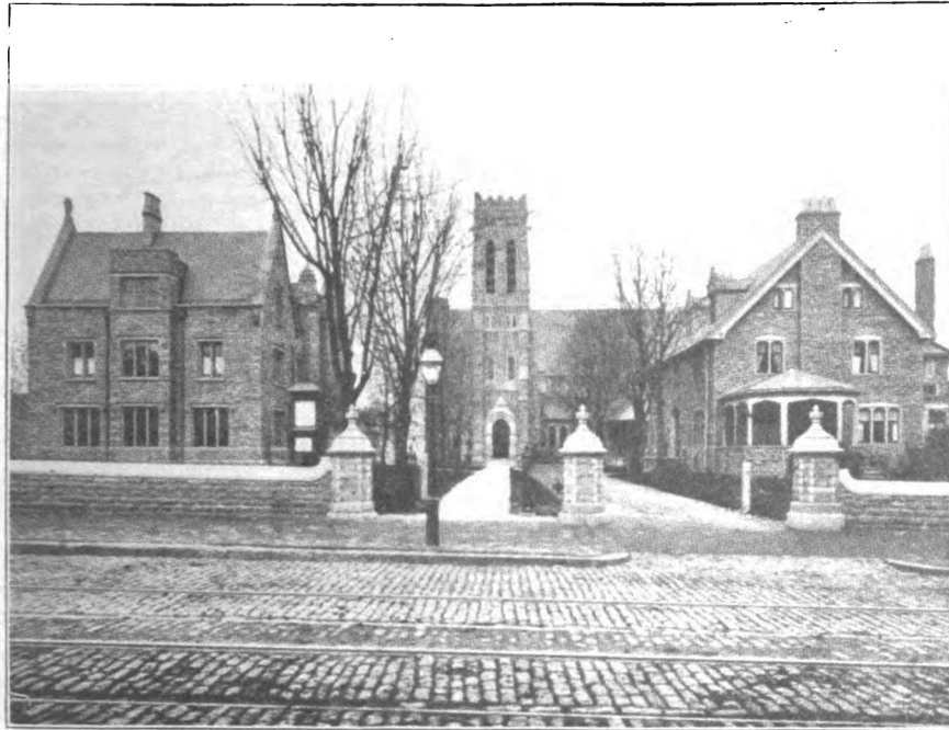
ST. LUKE'S CHURCH AND RECTORY AND ST. MARGARET'S HOME, GERMANTOWN, PA.
