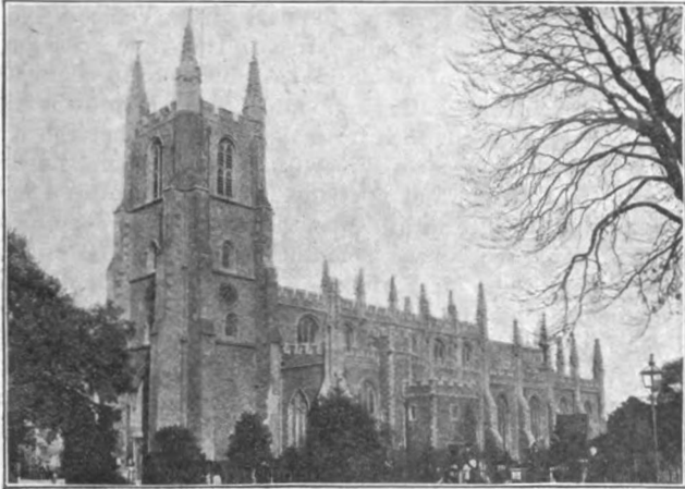
ST. JOHN BAPTIST CHURCH, CROYDON.
