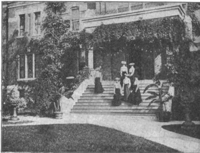
ST. MARY'S, MAIN ENTRANCE, SOUTH COURT.
