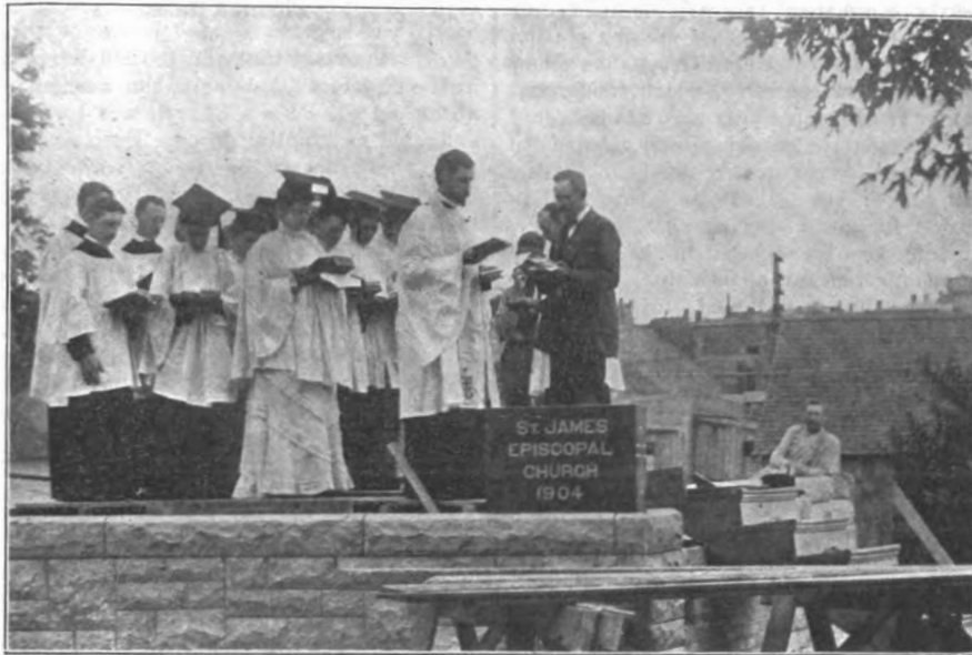
LAYING OF CORNERSTONE, ST. JAMES' CHURCH, MACON, MO.
