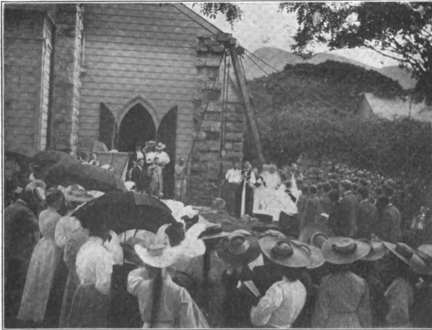
LAYING THE FIRST STONE OF ADDITION TO ST. ANDREW'S CATHEDRAL, HONOLULU.
