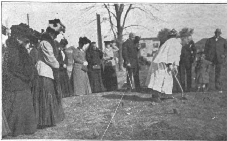
BREAKING GROUND FOR THE NEW ST. PAUL'S CHURCH, SAVANNAH, GA.
