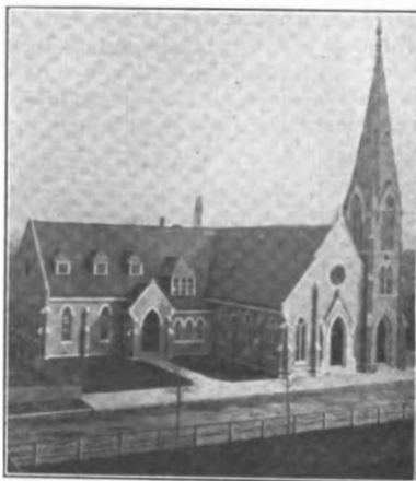
GRACE CHURCH AND PARISH HOUSE, HOPKINSVILLE, KY.
