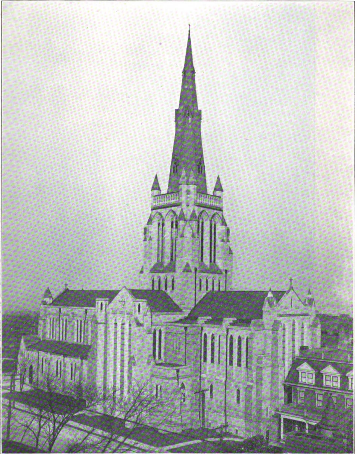
CALVARY CHURCH, PITTSBURGH, FROM THE SOUTH. [Illustrations from Photographs by R. W. Johnston.]
