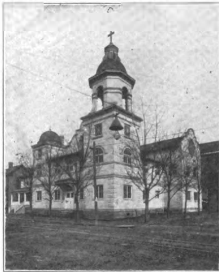
ST. ANDREW'S CHURCH, WHEELING, W. VA.
