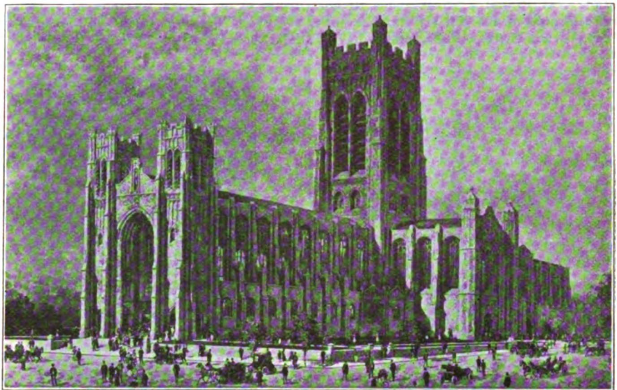
ST. JOHN'S CATHEDRAL, DENVER (IN COURSE OF ERECTION).
