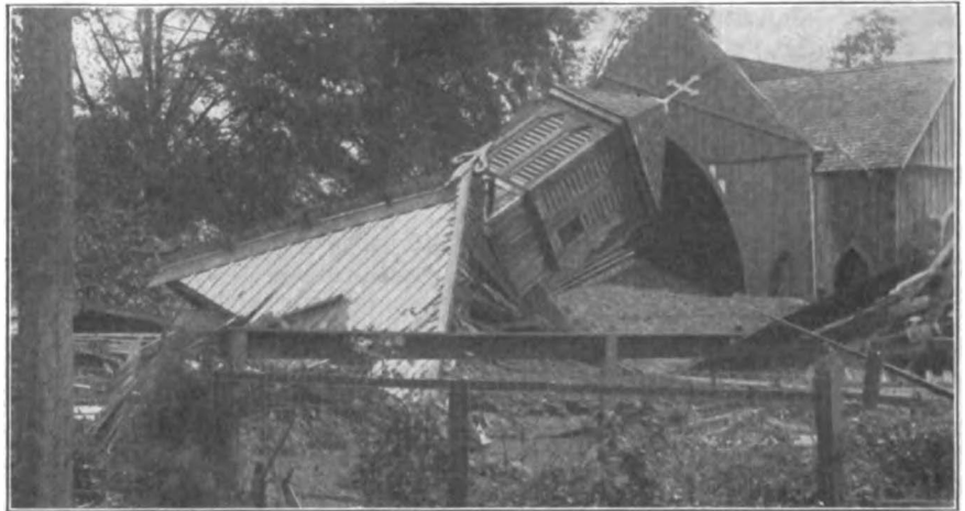
CHURCH WRECKED BY CYCLONE—CHURCH OF THE INCARNATION, AMITE, LA.
