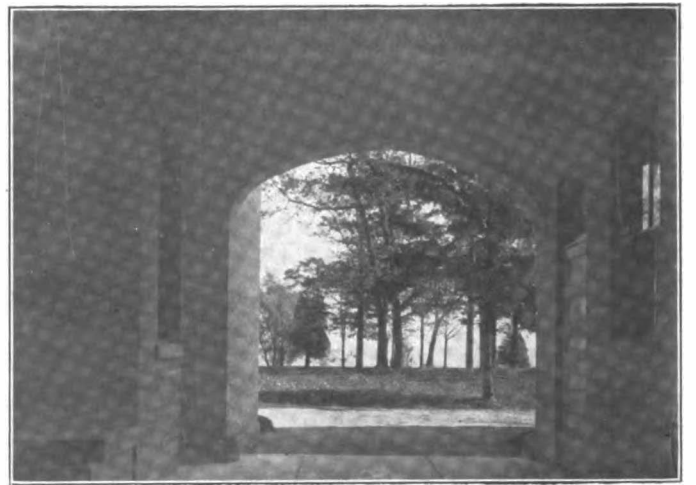
VIEW FROM THE ARCHWAY.
