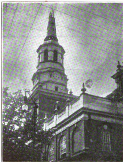
CHRIST CHURCH, PHILADELPHIA, SHOWING THE STEEPLE DAMAGED BY LIGHTNING.
