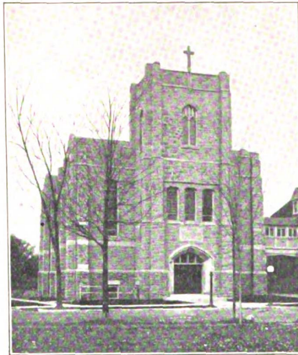
COLEMAN MEMORIAL PARISH HOUSE, CHURCH OF THE REDEEMER, SAYRE, PA.
