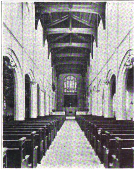
NAVE, LOOKING EAST. ST. MARK'S CHURCH, FRANKFORD, PHILADELPHIA.
