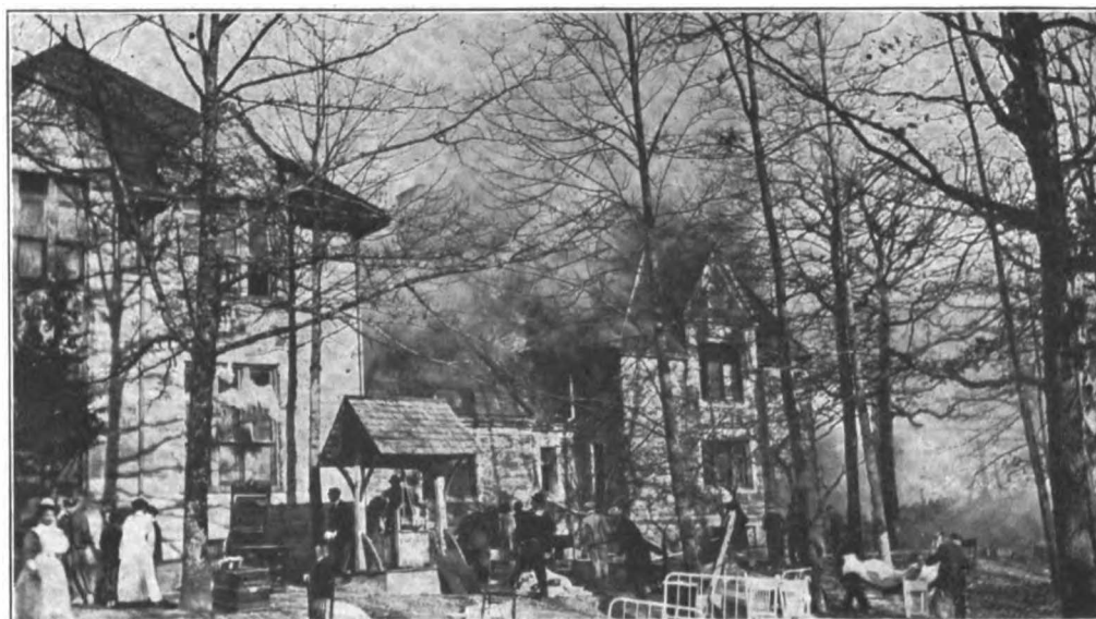
VIEW DURING THE FIRE.—HODGSON MEMORIAL HOSPITAL, SEWANEE, TENN.
