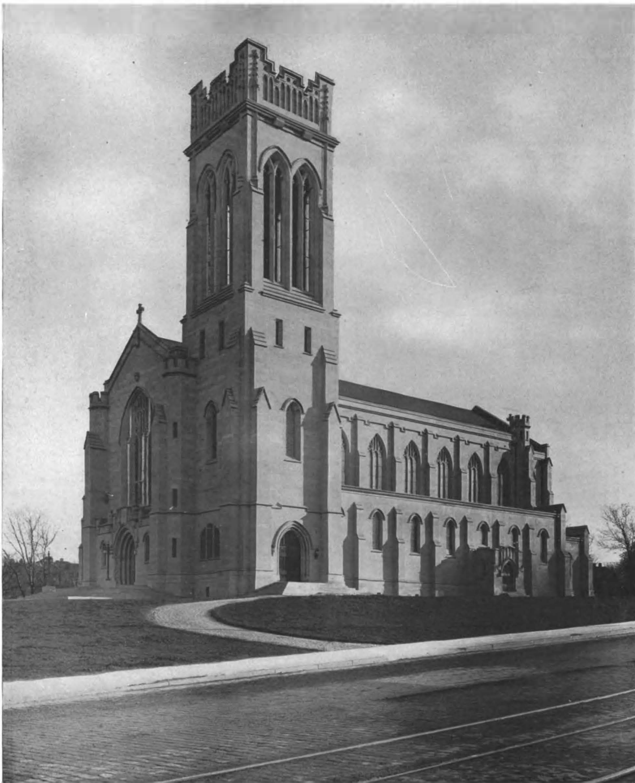
ST. MARK'S PRO-CATHEDRAL, MINNEAPOLIS. [By courtesy of "The Western Architect."]
