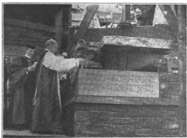
LAYING THE CORNERSTONE, INTERCESSION CHAPEL, NEW YORK [Showing Bishop Greer and the Architect, B. G. Goodhue, of the firm of Cram, Goodhue & Ferguson]
