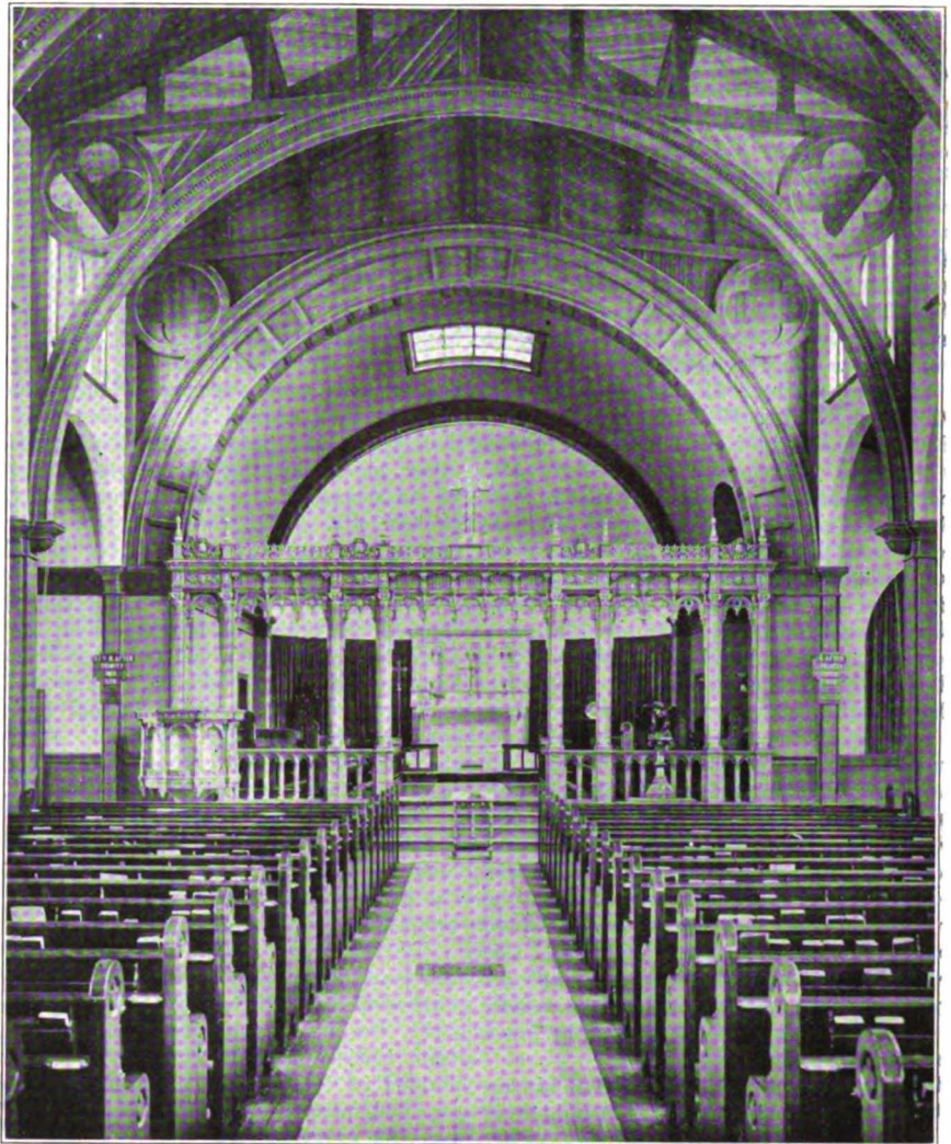
INTERIOR OF ST. MARK'S CHURCH, BERKELEY, CAL.
