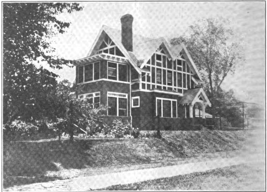
RECTORY OF THE CHURCH OF ST. JOHN BAPTIST, MINNEAPOLIS, MINN.
