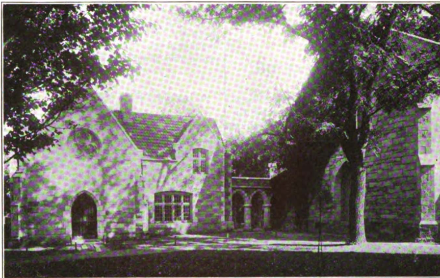
NEW PARISH HOUSE, CHRIST CHURCH Raleigh, N. C.
