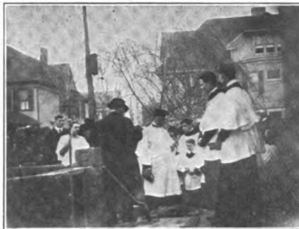
LAYING THE CORNERSTONE St. Jude's, Brooklyn
