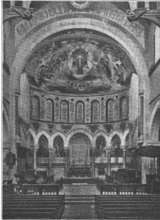
CHANCEL AND DOME Church of the Saviour, Philadelphia
