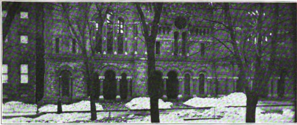
EXTERIOR VIEW. FRONT WALL OF CHURCH AND SUNDAY SCHOOL BUILDING
