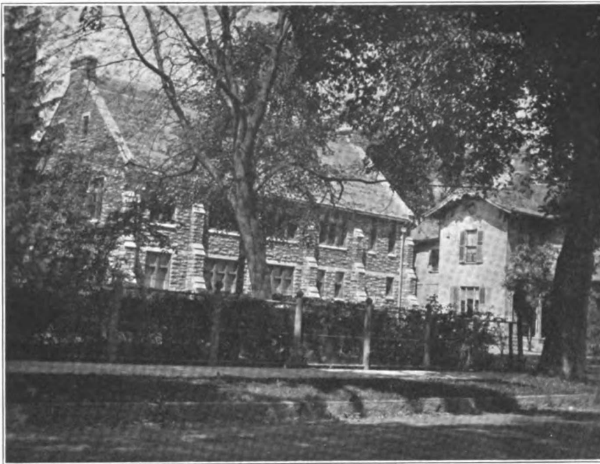
HOARD-HOWARD MEMORIAL PARISH HOUSE St. John's Church, Ogdensburg, N. Y.
