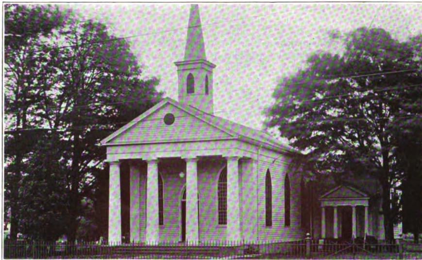
ST. JAMES' CHURCH AND PARISH HOUSE Piscatawaytown, N. J.
