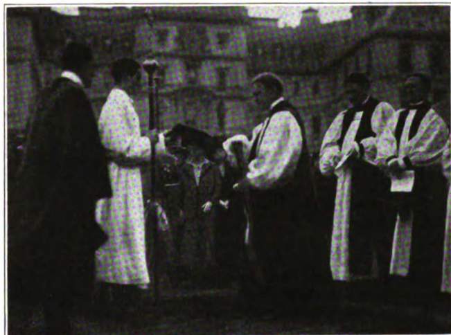
AT THE BREAKING OF THE GROUND FOR THE NAVE OF THE CATHEDRAL
