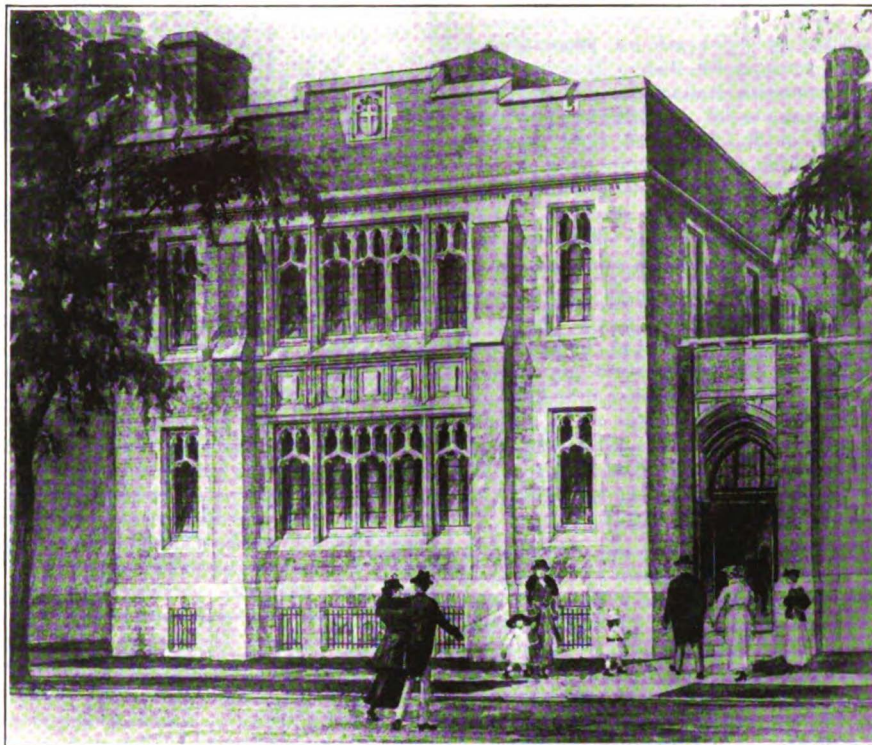
ST. MATTHIAS' PARISH HOUSE, DETROIT, MICH.
