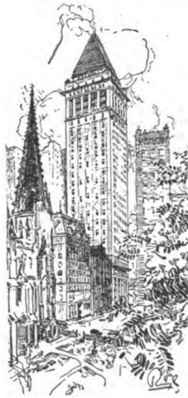
Bankers Trust Company Building
