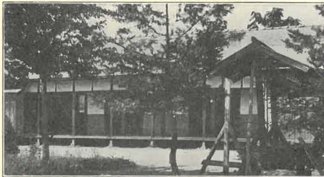
THE KINDERGARTEN CHURCH AT WAKAMATSU
