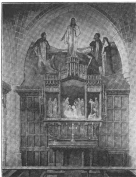
INTERIOR, HEWITT MEMORIAL CHAPEL, MINNEAPOLIS
