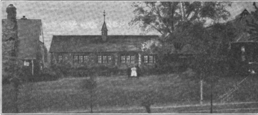
PARISH HOUSE, ROSELLE, N. J.
