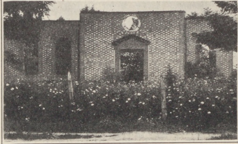
NORTH FARNHAM PARISH CHURCH WALLS BEFORE RESTORATION
