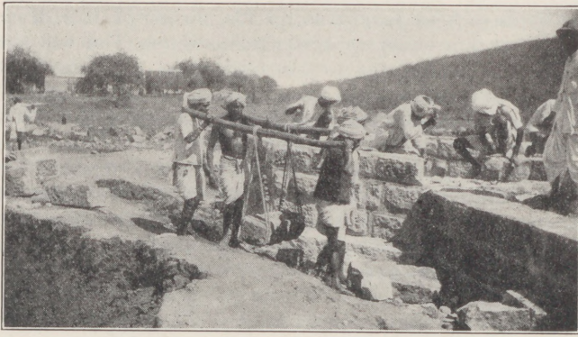
LAYING THE FOUNDATION FOR THE CATHEDRAL, DORNAKAL
