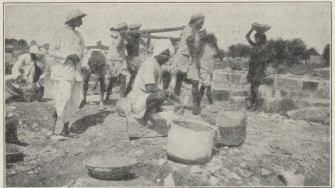
AT WORK ON THE BUILDING OF THE DORNAKAL CATHEDRAL
