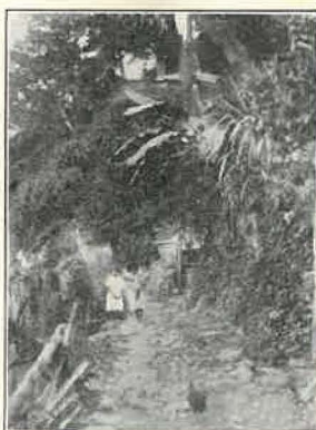
ROAD IN LUBON
