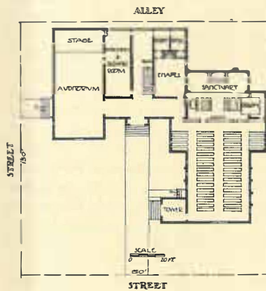
Figure 4 - Main Floor, Completed
