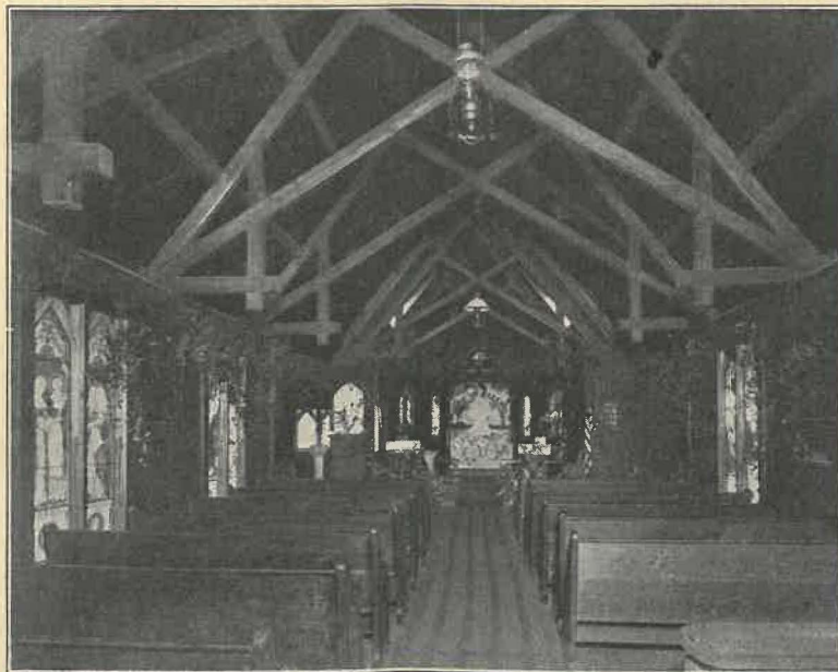
INTERIOR OF CHRIST CHURCH, FREDERICA, GA. Note the old kerosene lighting system
