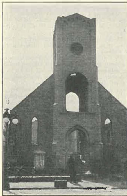
ST. PAUL'S CHURCH, LOCK HAVEN, PA.
