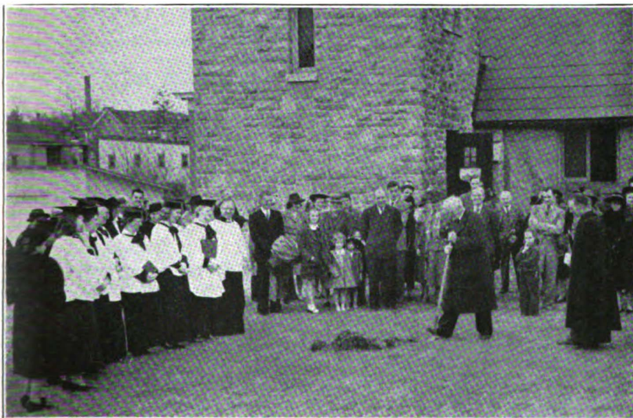
GROUND BREAKING: For a parish house which will be a student center.
