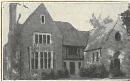
ST. FRANCIS HOUSE, MADISON, WIS.
