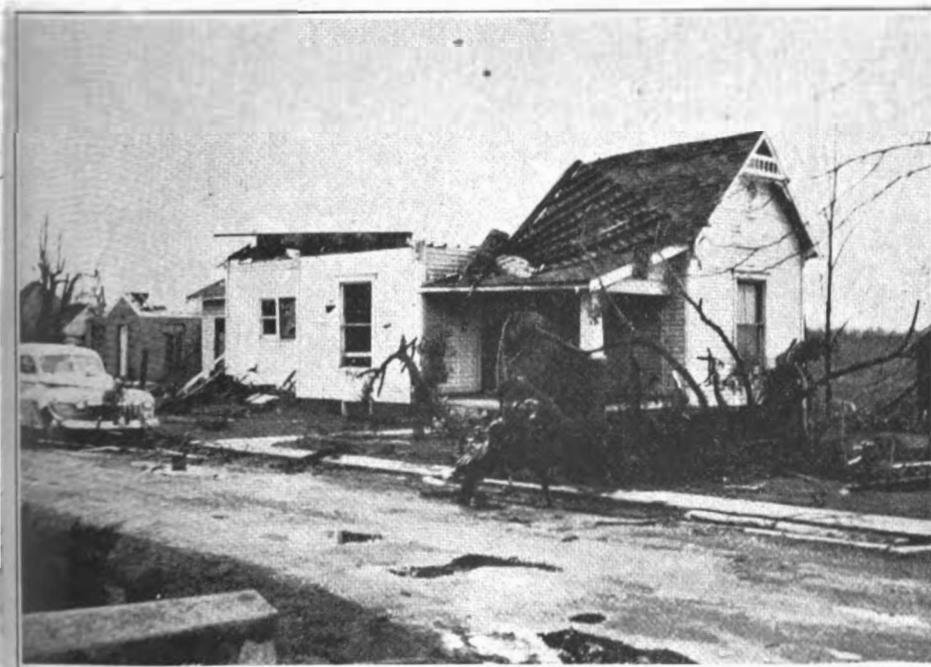
DEMOLISHED HOME OF DR. EDGAR C. CUMINGS.
