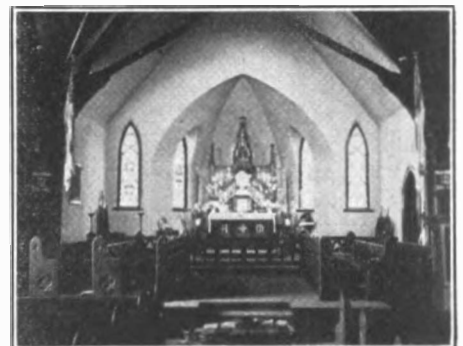
ST. JOHN'S CHURCH, NAPERVILLE
