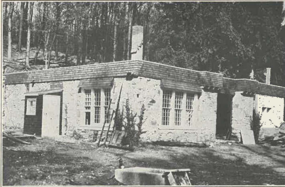
CHAPEL MADE FROM CARRIAGE HOUSE: Frame second story was unsafe, and therefore removed.
