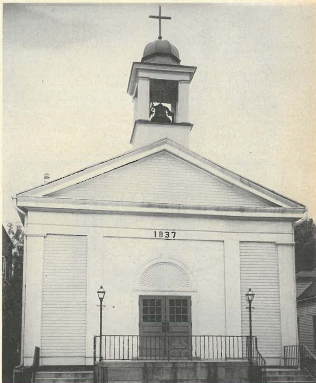
ST. JOHN'S CHURCH, CRAWFORDSVILLE, IND.
