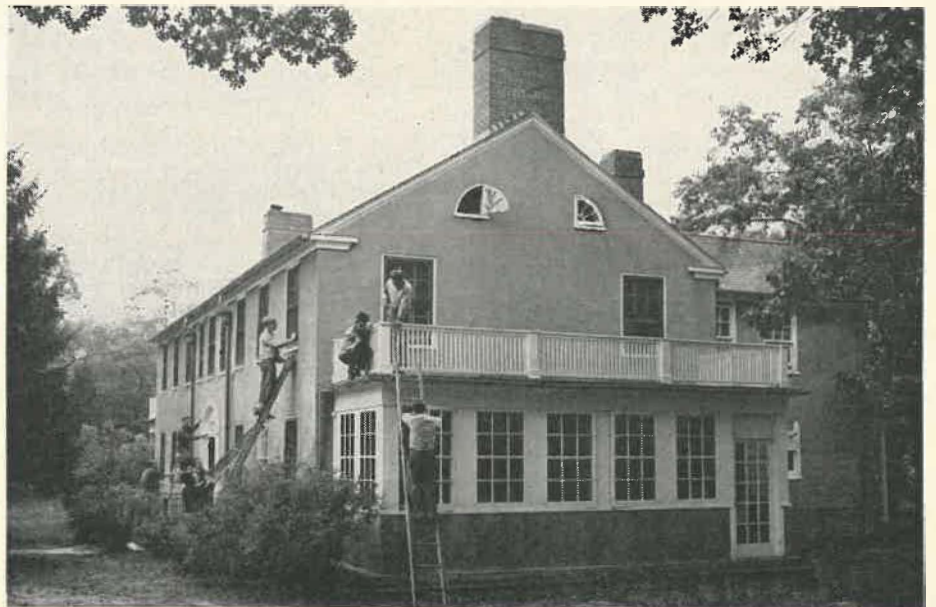
BROTHERS OF ST. JOSEPH repairing one of the diocesan center buildings.
