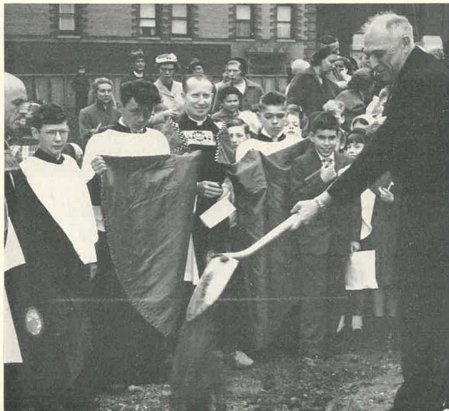
ST. LUKE'S GROUNDBREAKING: Continuation of a Policy.
